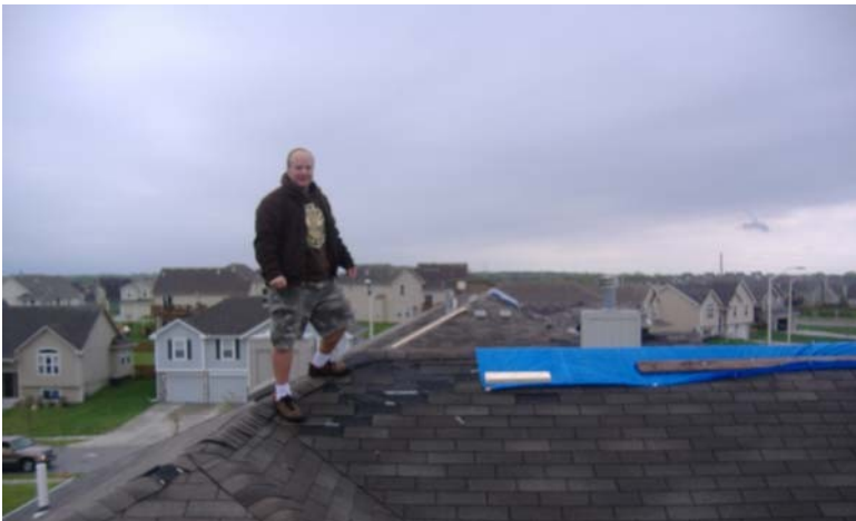
Making Repairs After a Thurse Passed Over Our House
